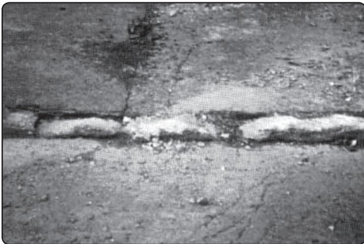
FIGURE 7: View of a completely deteriorated concrete curb.
