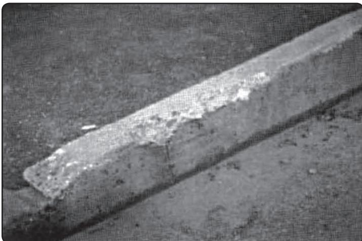
FIGURE 5: Concrete in the long run is susceptible to problems such as spalling.
