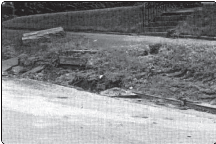
FIGURE 4: Due to its long life span, granite curb can be removed and reset to a new line or grade.
