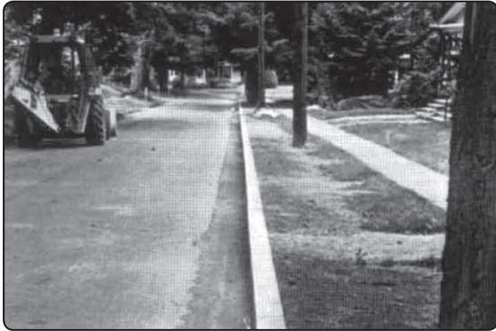
FIGURE 3: Modern machinery and methods produce granite curbs with neatly sawn tops and smooth split faces, adding to the aesthetic appearance of pavement.
