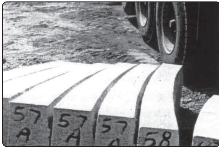
FIGURE 1: Standardized granite vertical curb (radius).
