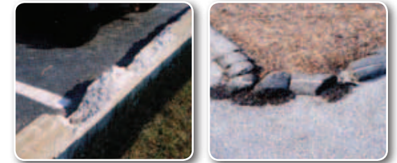
Concrete curb cannot survive even a short period if it is not backed up by soil. Berm always fails the snowplow test.
